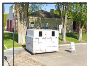
Herriman Fire Station 5928 W 13100 S
